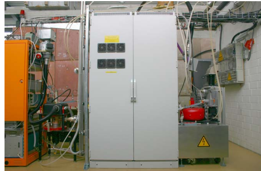
HoBiCaT transmitter: in the middle the power supply, right side the 10 kW klystron and left side the IOT prototype
