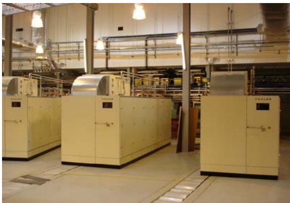
Power supplies feeding the IOTs
